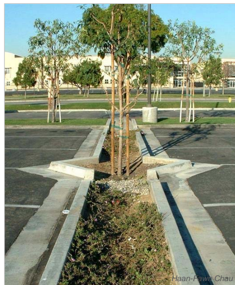
A vegetated swale with curb cuts in the parking lot of a shopping center at 8500 Firestone Blvd., Downey, CA.
