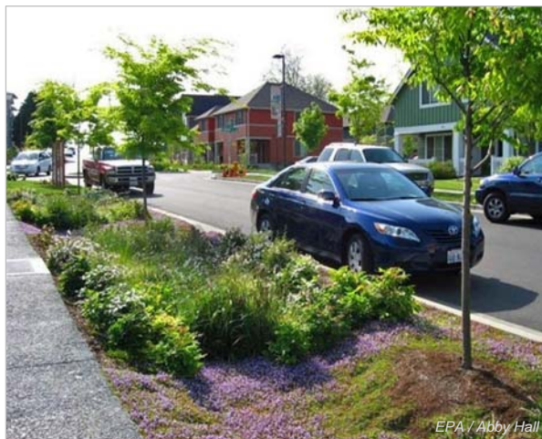
Seattle’s SEA Street (Street Edge Alternatives) project includes bioswales and permeable pavement.
